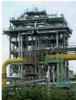
Surveying pipe geometries
